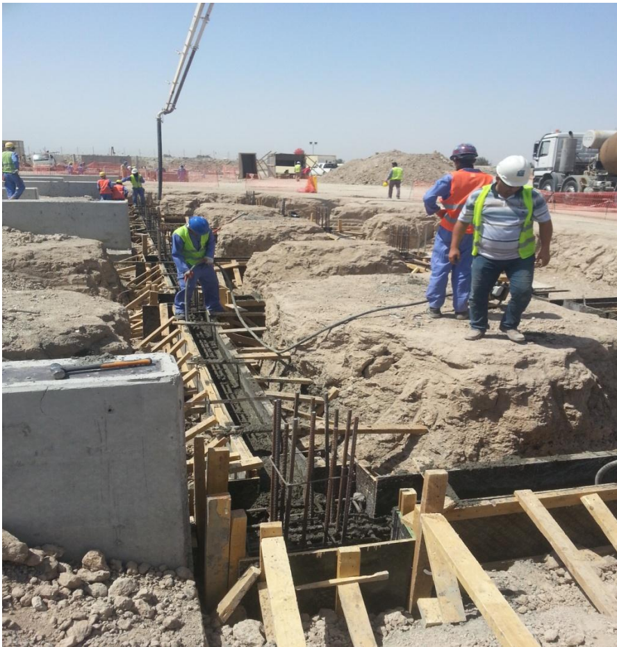
Concrete pouring for foundation
