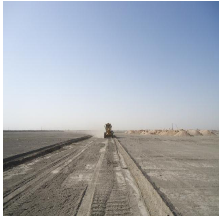
Grading and leveling road
