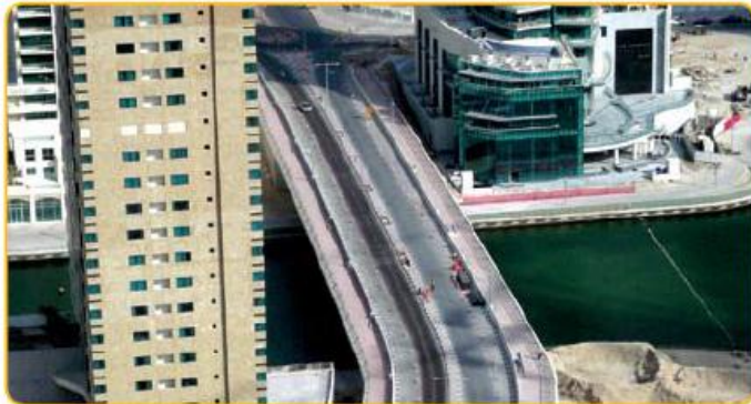
Improvement of Al Safouh Area Road Networks
