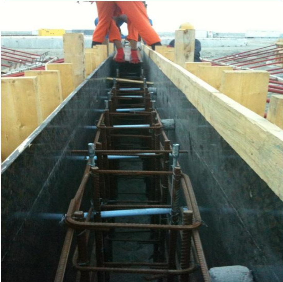
Rebar work for sleeper
