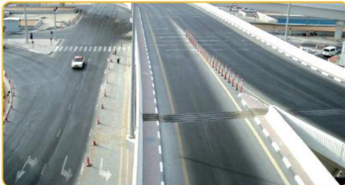
Al Ittihad Road Improvement
