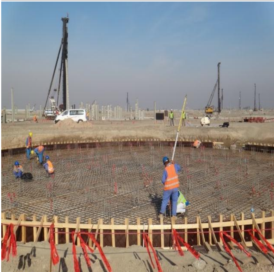
Concrete Pouring for Tank Foundation
