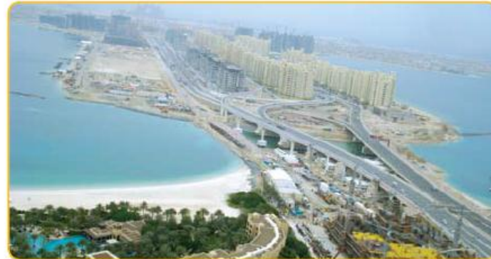
Palm Island Viaducts and Ramps
