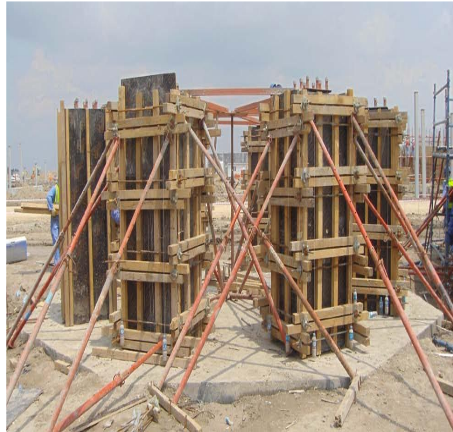
Form Work for Heater foundation pedestals
