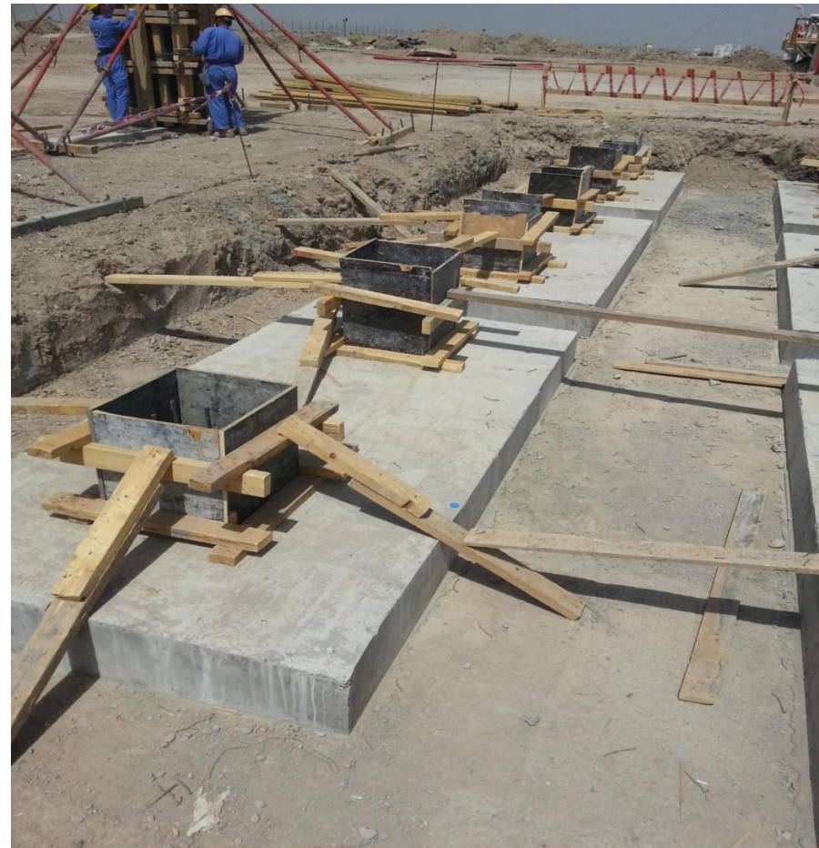
Form work for pipe rack
