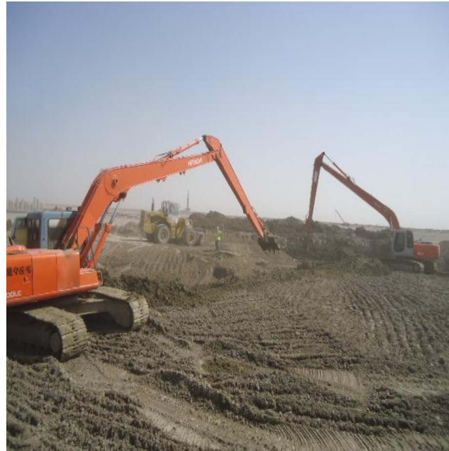
Excavations work for Tank Foundation
