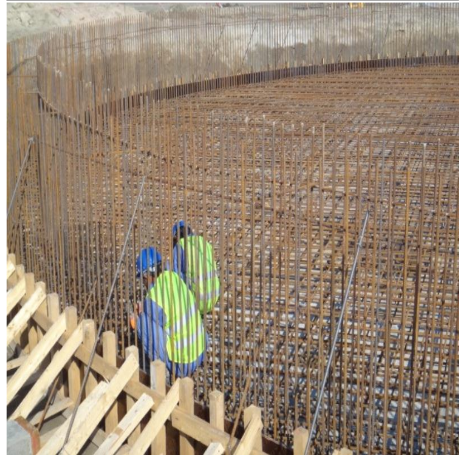
Dowels Rebar Work for Tank foundation
