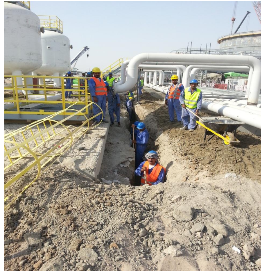
Manual excavation for pipe trench
