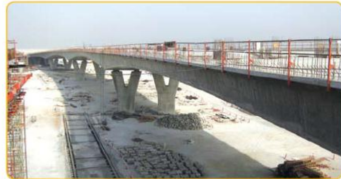
Palm Deira Access Bridge
