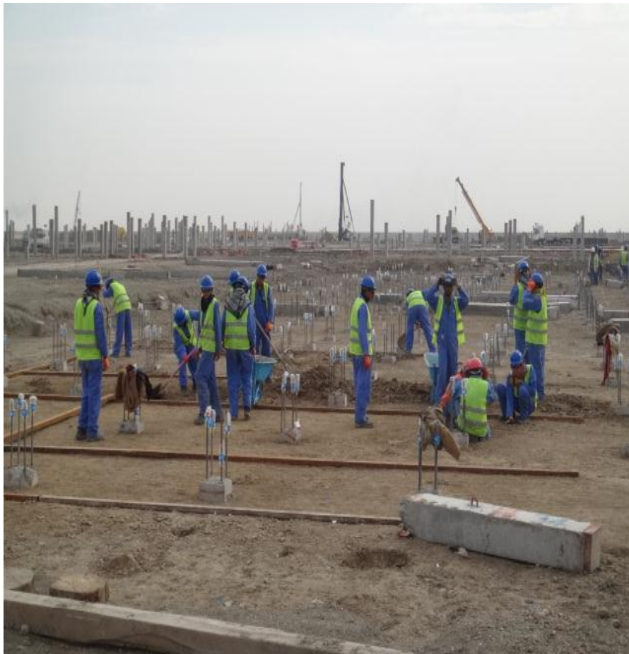
Leveling and preparing for lean concrete in cooling tower
