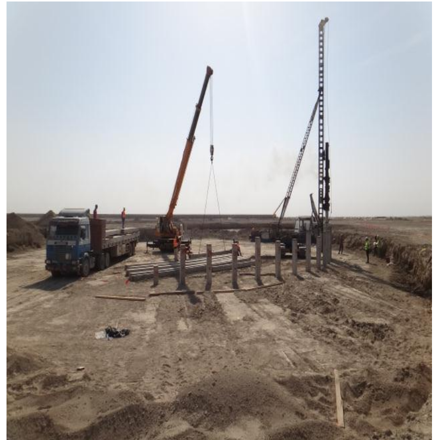
Driven piles in tank
