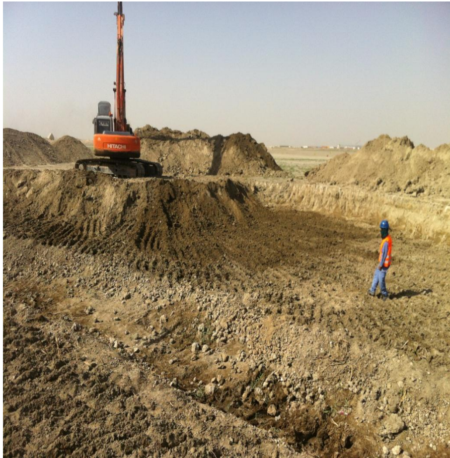
Excavations Work for Tank Foundation
