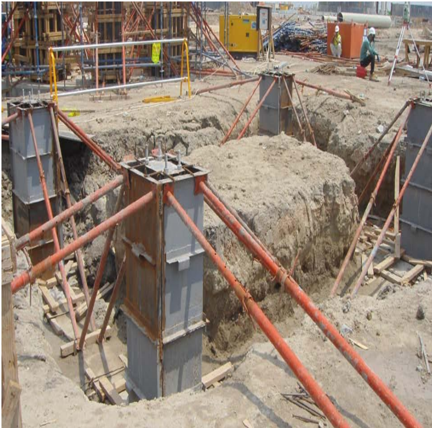
Metal form work for pipe rack pedestals
