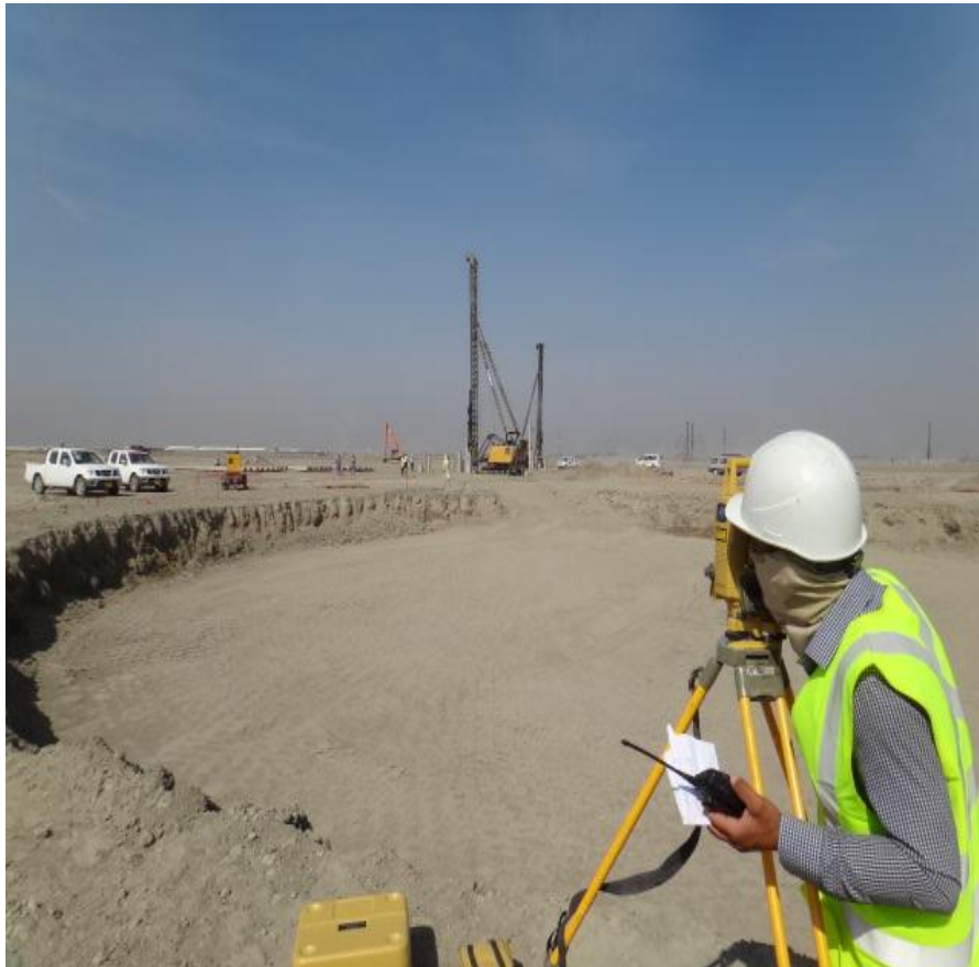
Survey Work for piles in tank foundation
